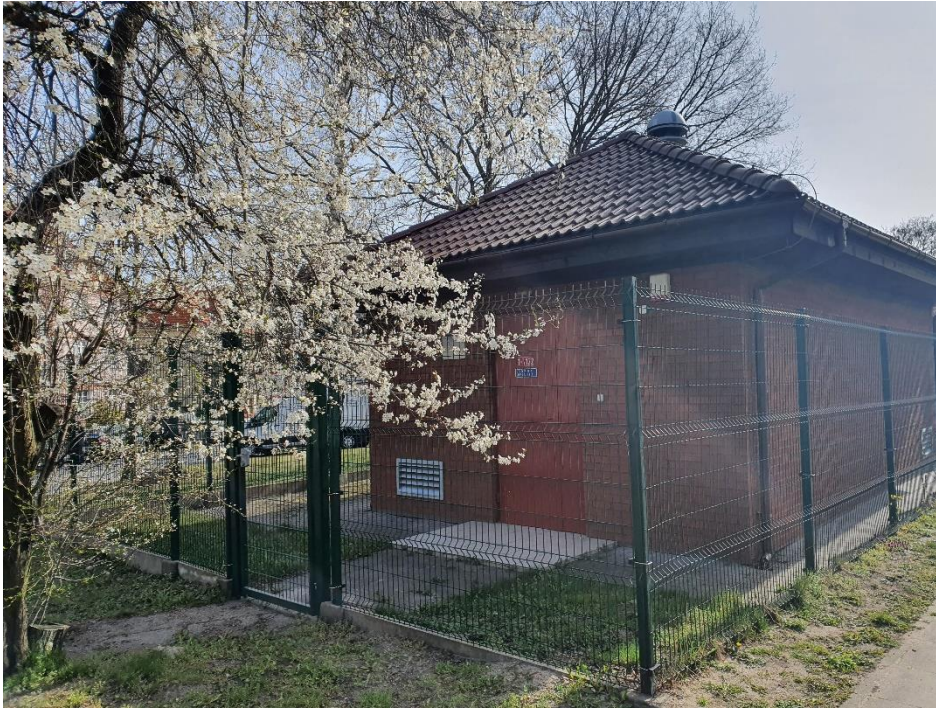
Figure 2. Sopot Reja substation
