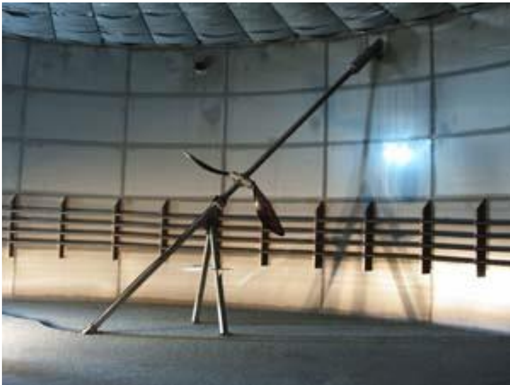
Figure 12. Mechanical agitator inside the fermentation chamber ( www.stallkamp.pl )
