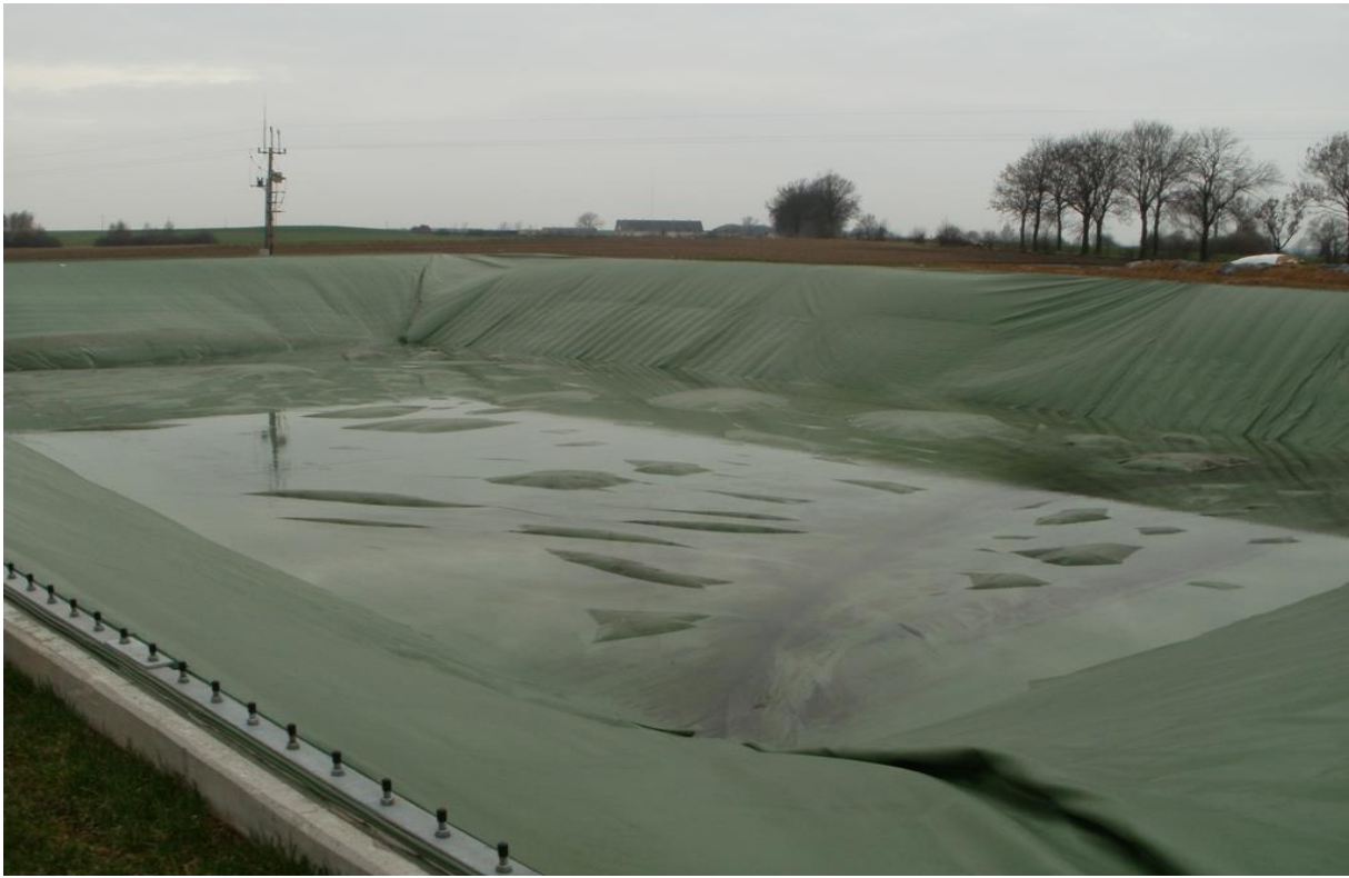
Figure 13. A lagoon in the area of an agricultural biogas plant (ph. Z. Ginalski)
