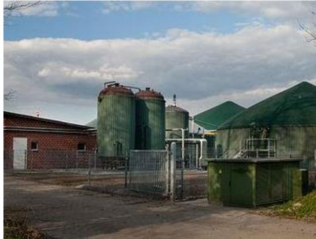
Figure 8. Substrate storage in a biogas plant Photo: C. Eckhardt, Wikimedia cc0 1.0
