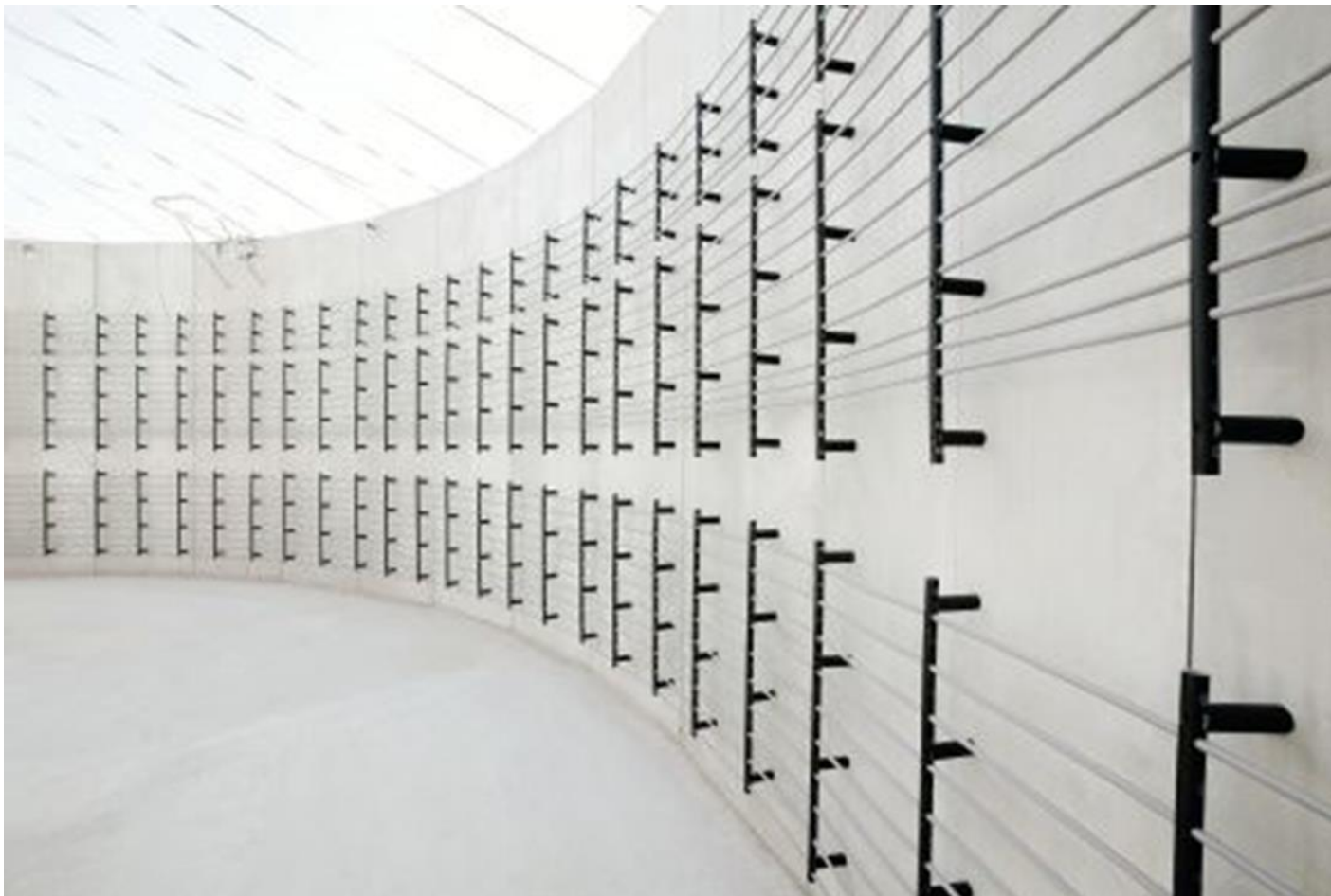
Figure 11. Heating pipes inside the fermentation chamber ( globenergia.pl )
